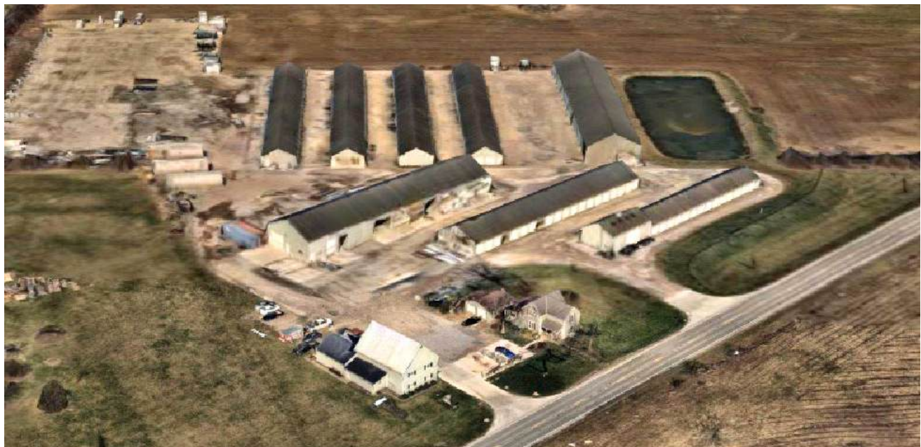
Northwest Building Resources and Storage
